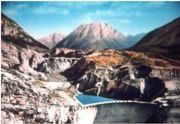
Figure 1.1b: During the filling of the Vajont reservoir the toe of the slope on Mount Teto was submerged and this precipitated a slide. The mound of debris from the slide is visible in the central part of the photograph. The very rapid descent of the slide material displaced the water in the reservoir causing a 100 m high wave to overtop the dam wall. The dam itself, visible in the foreground, was largely undamaged.
