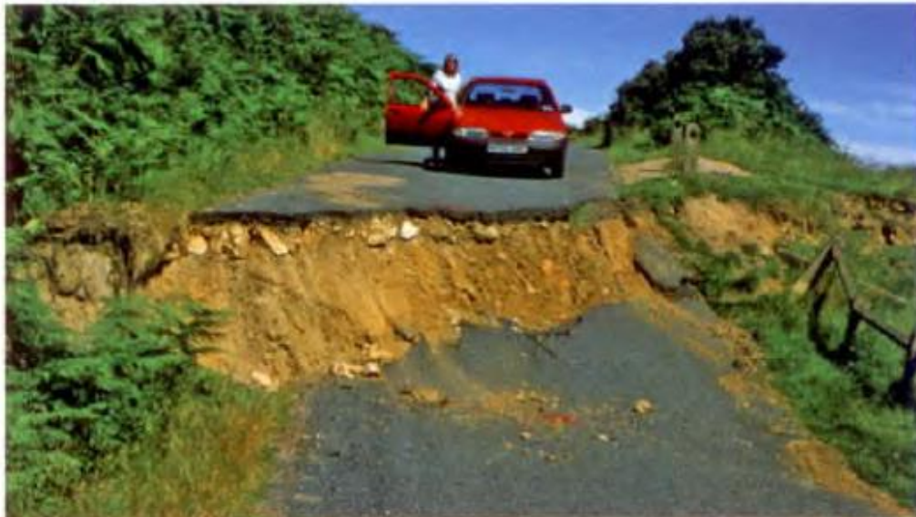
Head scar of a rotational slide breaks a road in Yorkshire.
