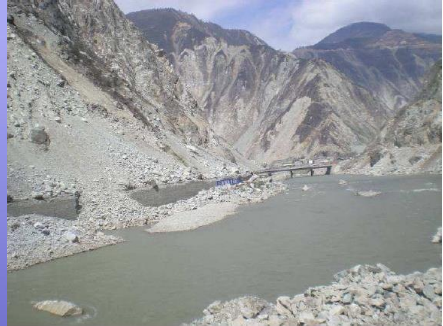
Fig. 6: Traces of rockfalls along valley and blockage of access roads on the right bank (Wenchuan earthquake)
