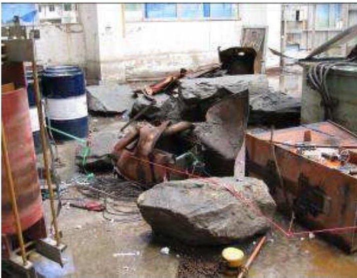
Fig. 5: Effect of rockfalls on powerhouse of the Shapai arch dam caused by the 2008 Wenchuan earthquake, Wall and roof punctured by high-velocity rocks (top) and electro-mechanical equipment damaged by rocks (bottom).
