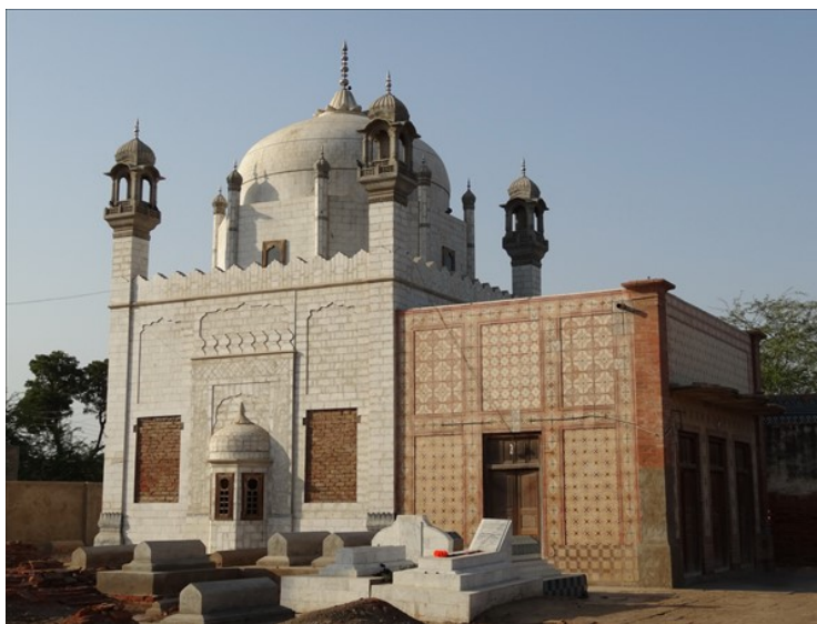
The Tomb of Pir Muhammad Ashraf Shah Quraishi after renovation
