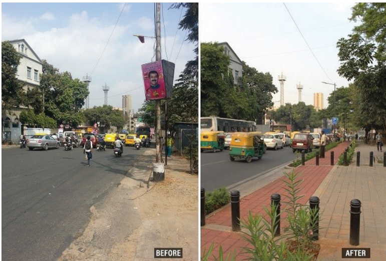
Figure 5.29: Sidewalk in Bengaluru, Redesigned into a Wide, Continuous, Protected Sidewalk with Fixed Bollards to Prevent Motor Vehicles from Encroaching onto the Pedestrian Space
