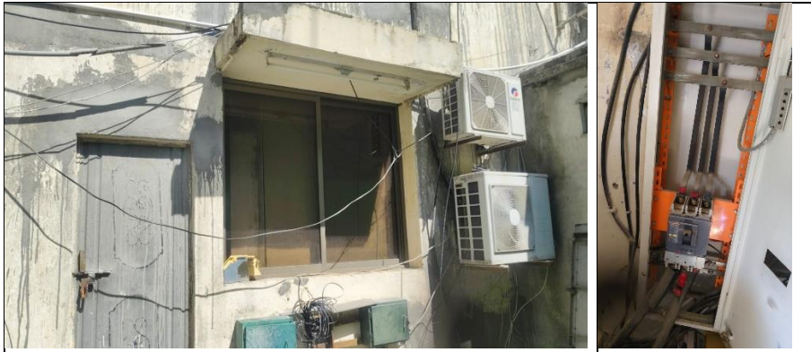
Control Room for Main Building
