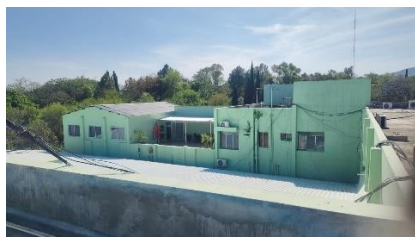
Cable Routing Towards Main Building – Ground Floor
