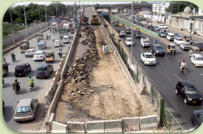
Fig. 2. Drigh Road Flyover Being Repaired
