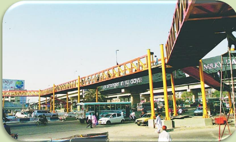
Fig. 3. Overhead Pedestrian Bridge in Karachi
