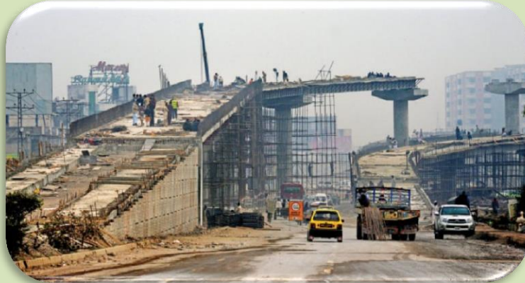
Fig. 1. Disruption Caused by the Construction of a Flyover in Peshawar
